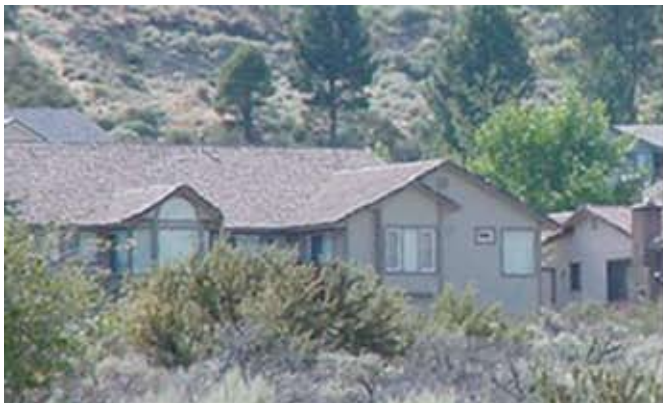
Prior to the fire, this homeowner changed the roof material from wood shakes to fire-resistant tiles and reduced the amount of flammable vegetation surrounding the home. These pre-fire activities helped this house survive the fire.
