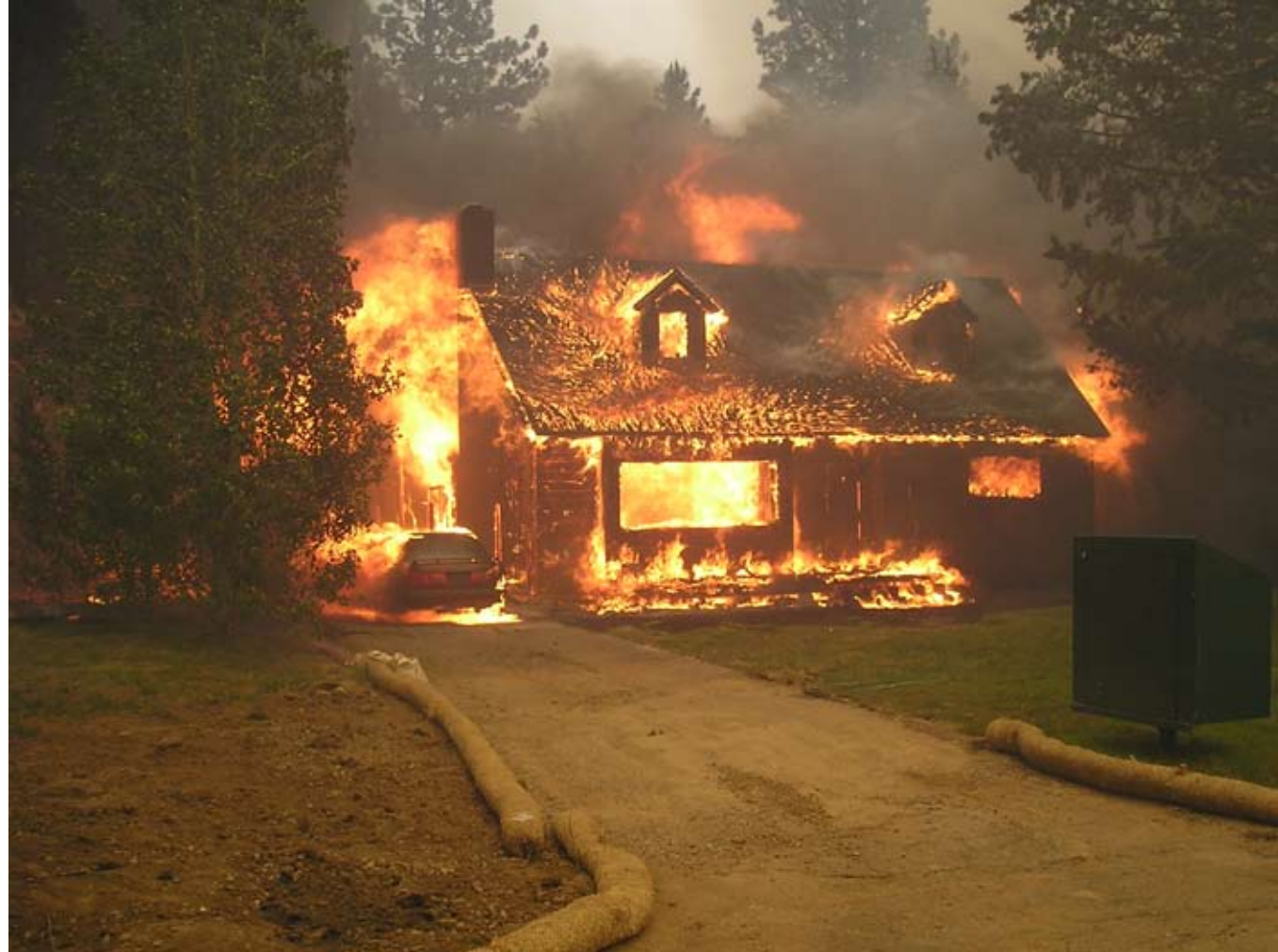
The 2007 Angora Fire destroyed 242 homes and damaged 35 others. The presence of unburned vegetation surrounding this house suggests a burning ember landed on something easily ignitable on or immediately adjacent to the home.
