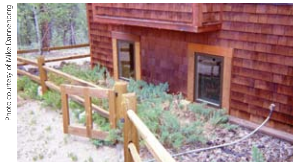
During a wildfire, airborne embers may land and accumulate in the area next to the house. Avoid using combustible materials, such as wood mulch, and flammable plants, such as juniper, within 5 feet of the home.
