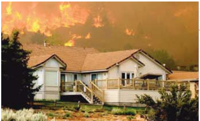
Prior to the fire, this homeowner changed the roof material from wood shakes to fire-resistant tiles and reduced the amount of flammable vegetation surrounding the home. These pre-fire activities helped this house survive the fire.
