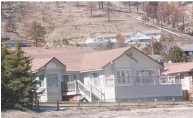
Prior to the fire, this homeowner changed the roof material from wood shakes to fire-resistant tiles and reduced the amount of flammable vegetation surrounding the home. These pre-fire activities helped this house survive the fire.
